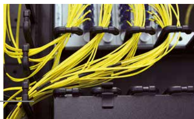
Cable clips, known as L-fingers, guarantee optimum protection against bending and kinking
